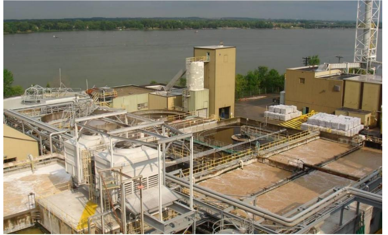
Essity plant in Menasha, Wisconsin.
